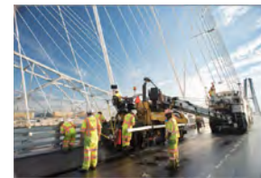
Mario M. Cuomo Bridge
