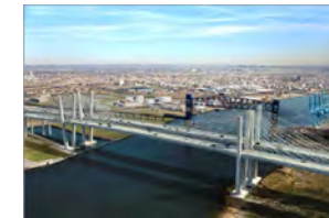
New Goethals Bridge
